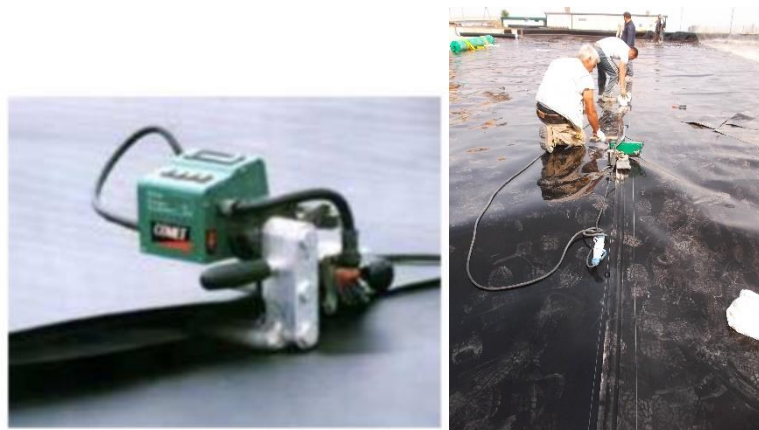
Figure 1: HDPE welding
