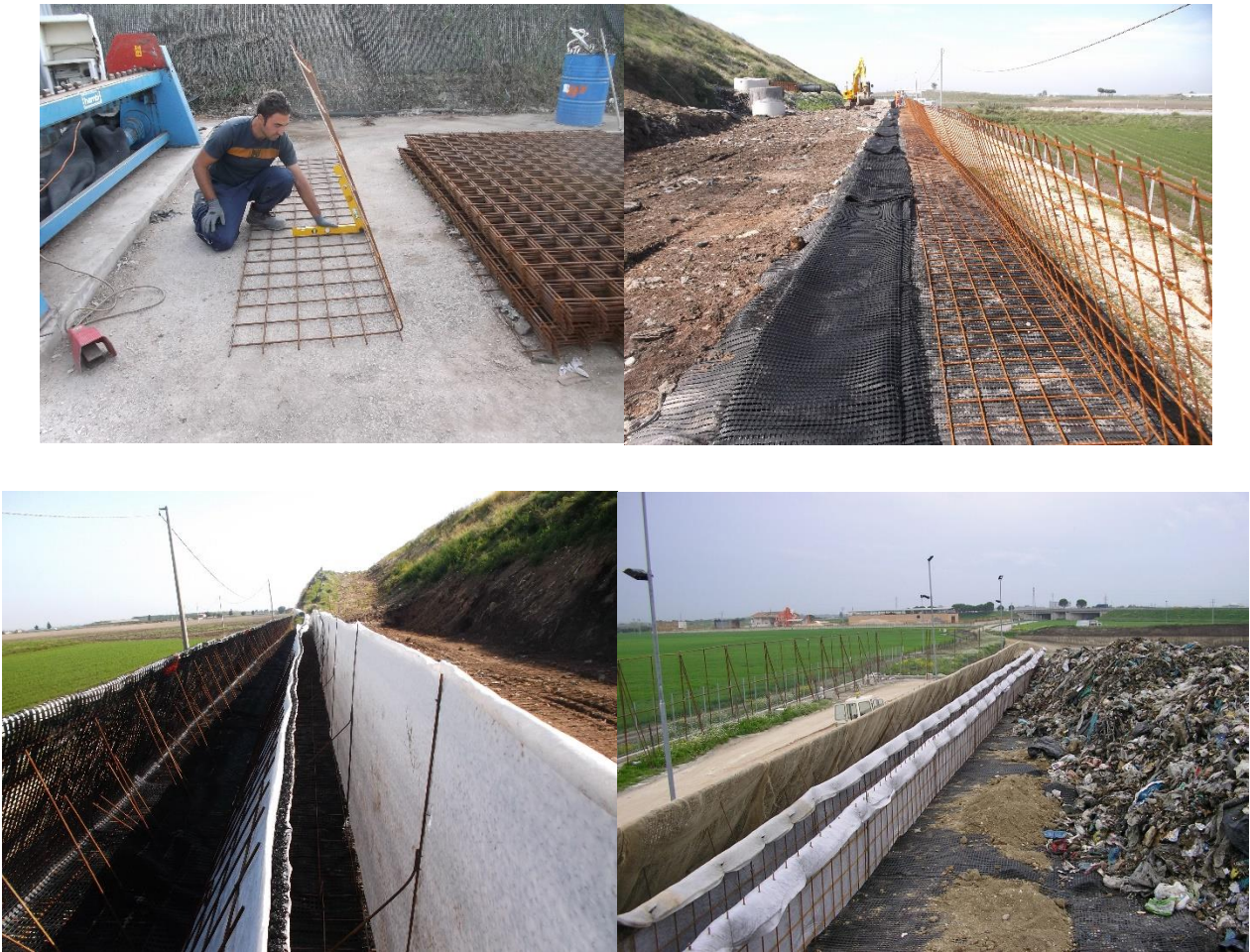
Figure 3: Construction phases of the retaining structures for waste
